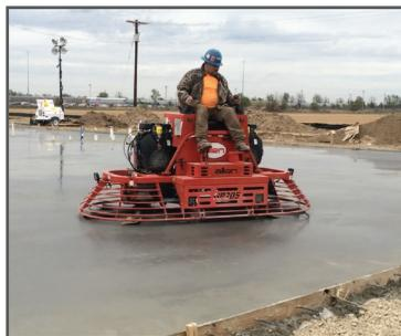
The HP205 riding trowel, features twin 37 hp Kohler EFI gasoline engines. These machines are workhorses built for concrete professionals to deliver maximum horse power with electronic fuel injection. Utilizing torque converter clutches, they provide excellent low speed torque for low speed float panning and superior high rotor speed for finishing concrete.
