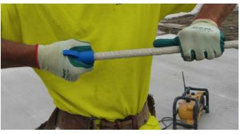
LOAD the FinCap in the driver an insert the mounting structure at the established location
