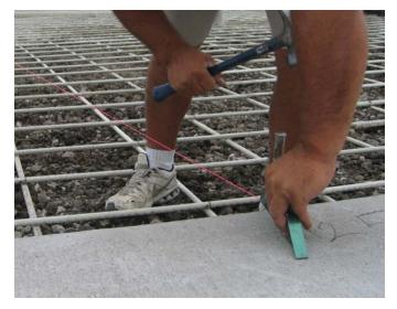
DETERMINE the finished elevation of concrete with a laser or string line
